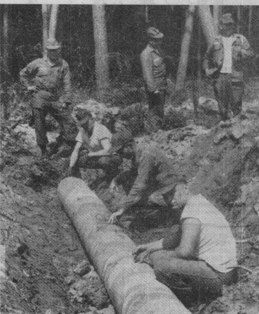
Men of 317th Engr Bn's Co D rest after laying parts of a drainage pipe for the storage area.
